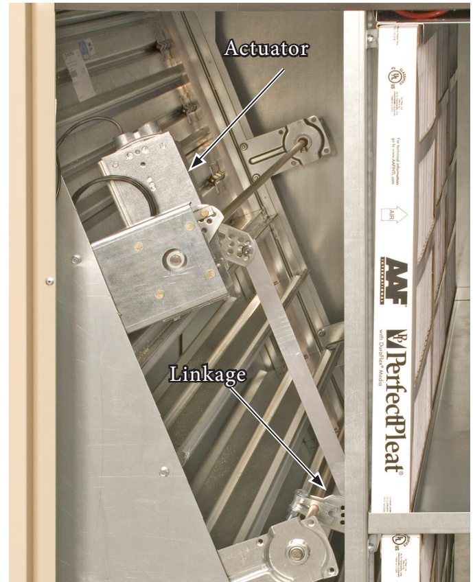
Figure 12: Damper Assembly
